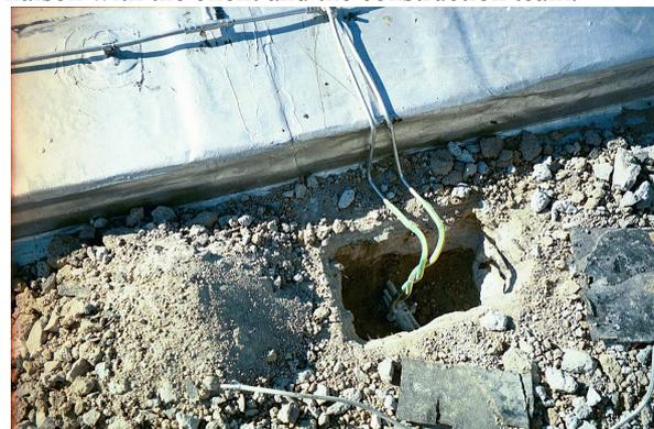
*Figure 5. Illustration of typical bonding of an air termination conductor to rebar on an existing structure. Sealing of bonds was given particular attention. The large hole was through non-structural cement screed (to then*
