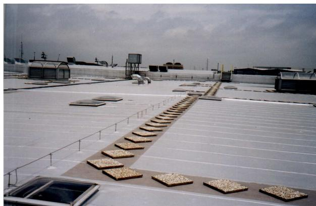
*Figure 1: Illustration of elevated horizontal air termination conductors*
