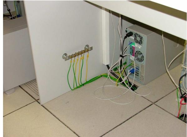
*Figure 4. This illustrates typical bonding between discrete servers and the access floor (whose galvanic continuity was ensured). Bonding was implemented via local bonding bars for maintenance convenience.*
