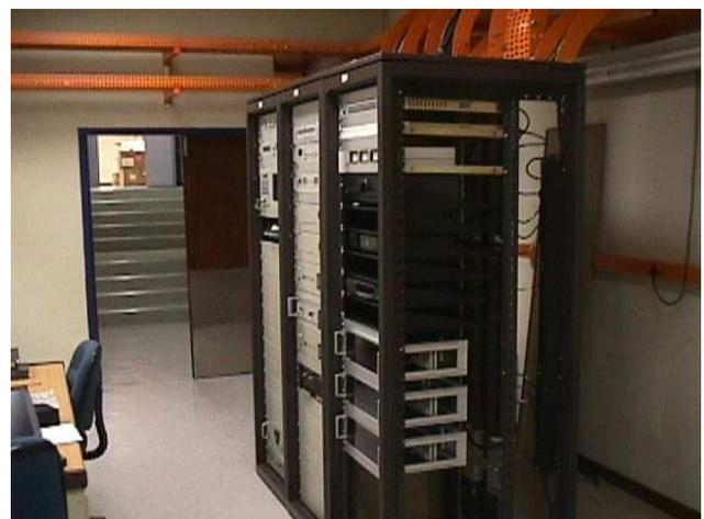
*Figure 3: Example of equipment installation. Note orange cable trays utilised for local equipotential bonding after their galvanic continuity was ensured.*
